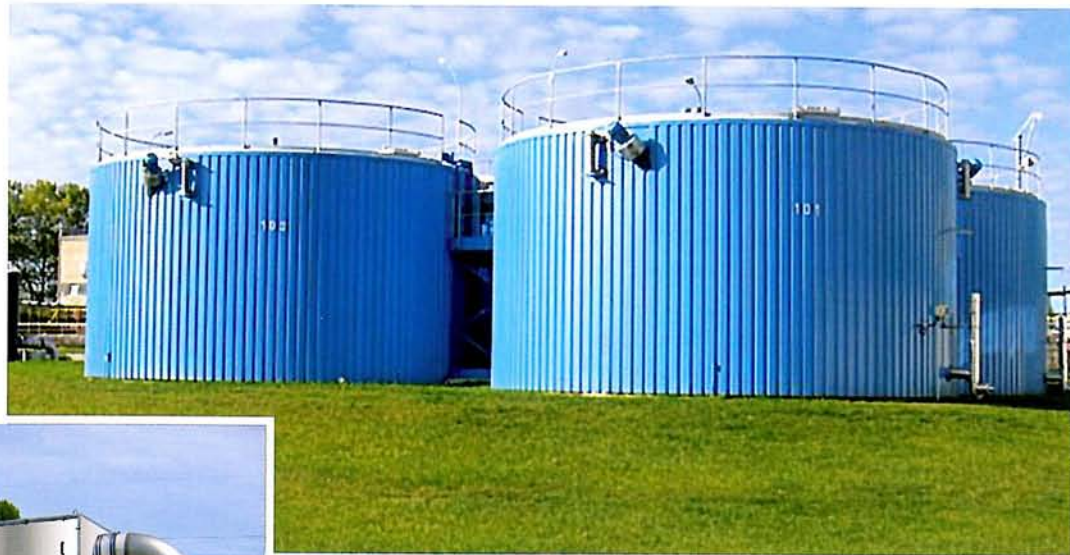
ATAD plant in Poland for a total population of 67,500 (3.57 MGD)
