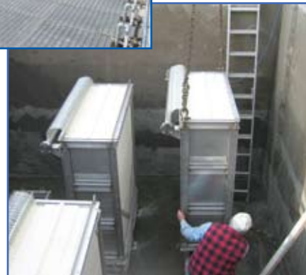
Installing the MBR units.
