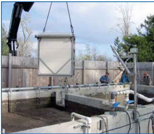
A SaniBrane® module being installed in a concrete tank.
